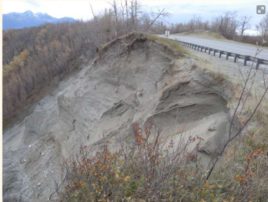
Unstable soil slope on Glenn Highway, MP 49.7 . Total USMP score is 518.
